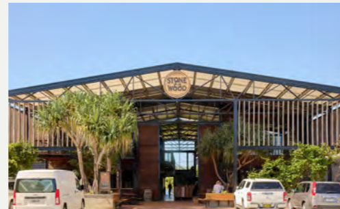
100 Centennial Cct, Byron Bay NSW. 350m.
