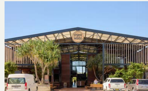
100 Centennial Cct, Byron Bay NSW. 350m.
